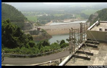
**PUMPING WATER TO UPPER DAM DURING LEAN HOURS (LOW COST POWER)**
